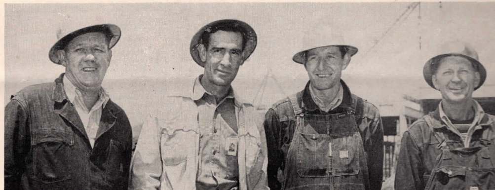
SHIPWRIGHTS . . . Erection Squads A & B
