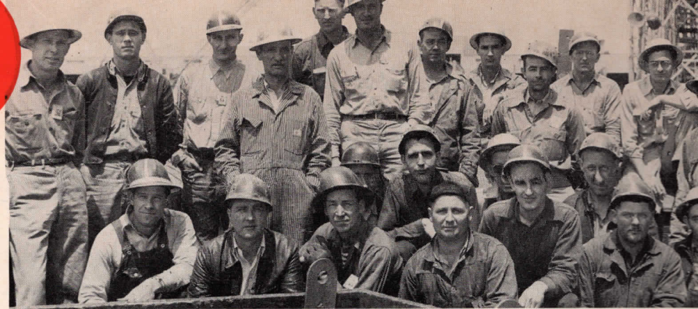
WELDERS . . . Erection Squads A & B, Shell and Foundations
