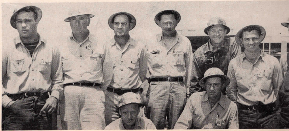
FLANGERS & CHIPPERS . . . Erection Squads A & B
