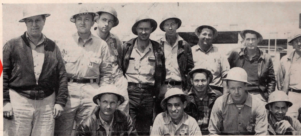
SHIPFITTERS . . . Erection Squads A & B and Foundations
